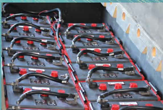
Electricity from the solar panels passes through wall-mounted inverters to a bank of 6-volt batteries, which store enough energy to power the house for up to three days.
